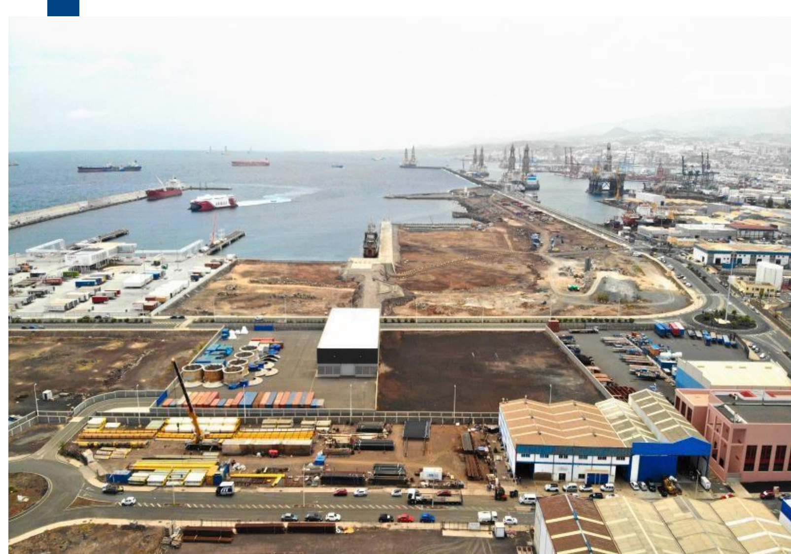
Zona Franca Las Palmas Port, Gran Canaria 15.000 m2 Free Trade Zone Mechanical and Hydraulic Workshops OCTG and logistic Yard
